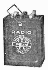
The Willard Al-Rubber Radio 'A' Battery has a one-piece rubber case—Threaded Rubber Insuation—special Radio plates.
